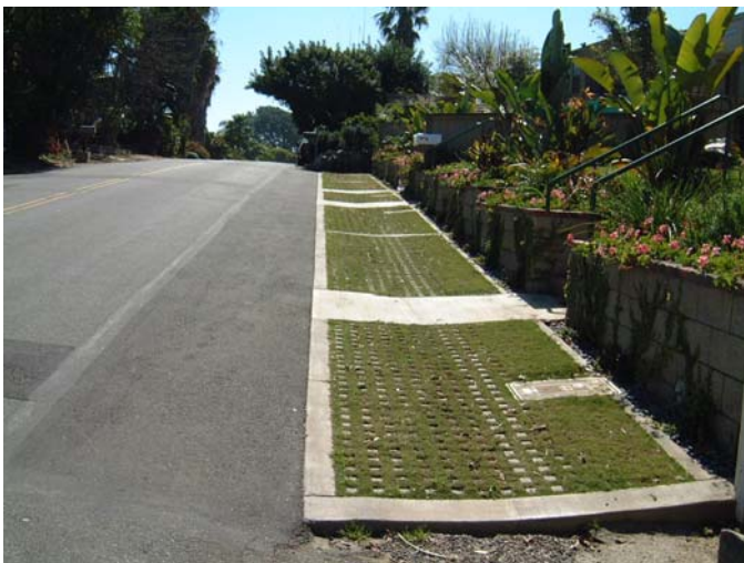
Photograph: City of Encinitas, Roadside GrassCrete parking
