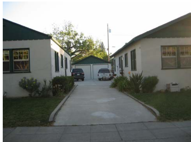
Photograph Courtesy of EOA, Inc.
