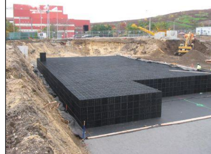
Underground detention tank Source: www.webtecgeos.com
