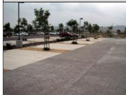
Permeable Pavement Source: Geosyntec Consultants
