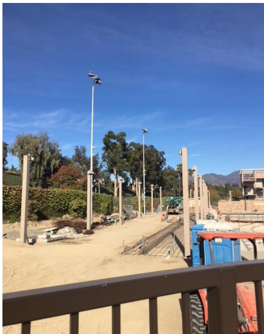
Grand Stand Shade Structure Columns
