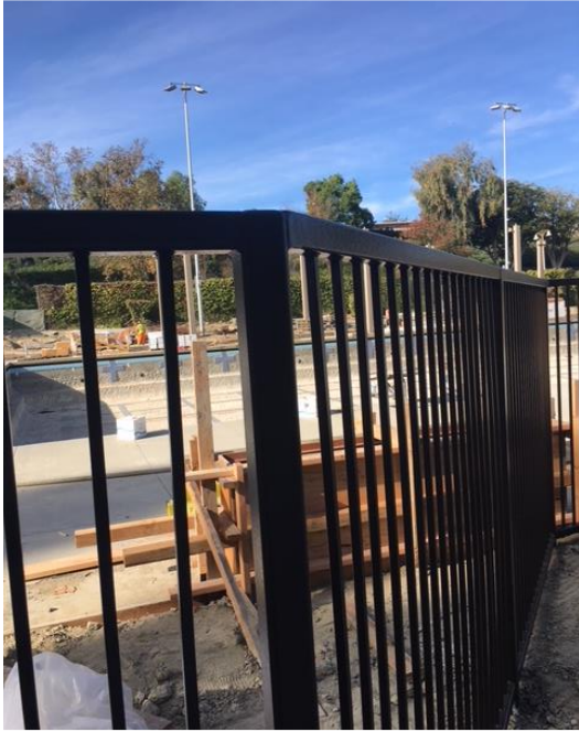
Perimeter Fence Installed/Painted
