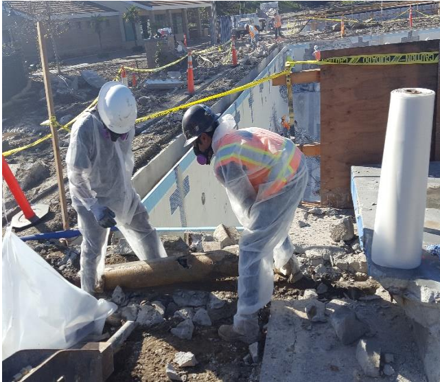
REMOVAL OF TRANSITE PIPE
