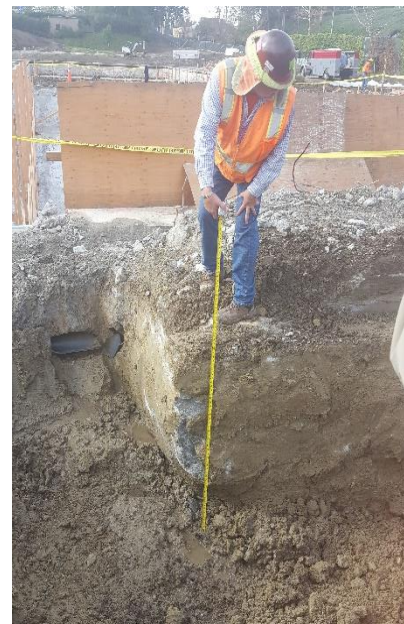
MASSIVE CONCRETE FOOTING UNDER 1 METER PLATFORM
