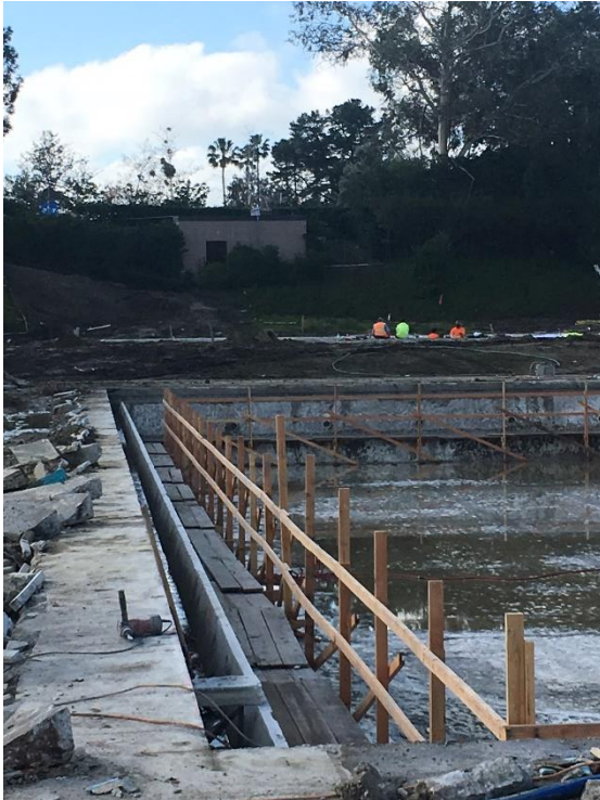
SCAFFOLDING BUILT AND GUTTER AND LIP EXPOSED
