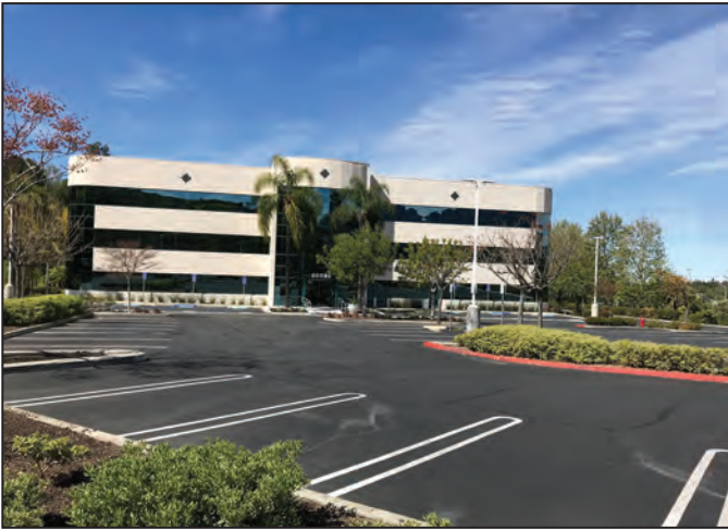
1. View looking from parking lot to Saddleback Church office building.
