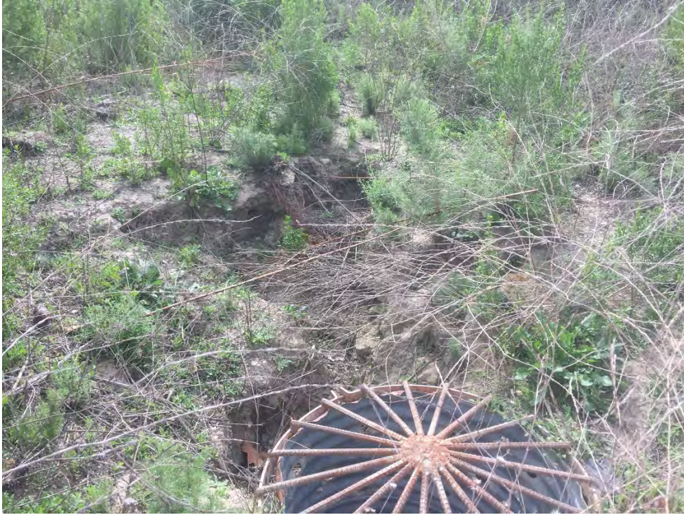
Photo 7: Drain at the end of Feature B; facing south.
