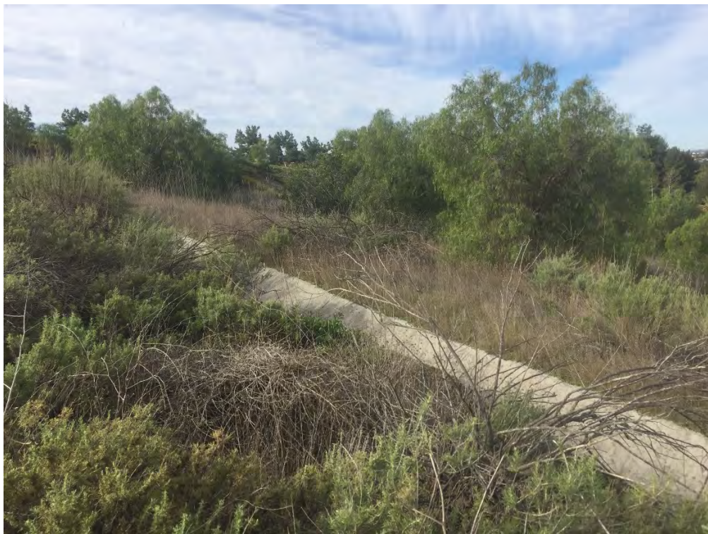
Photo 6: Feature B (concrete v-ditch); facing west.
