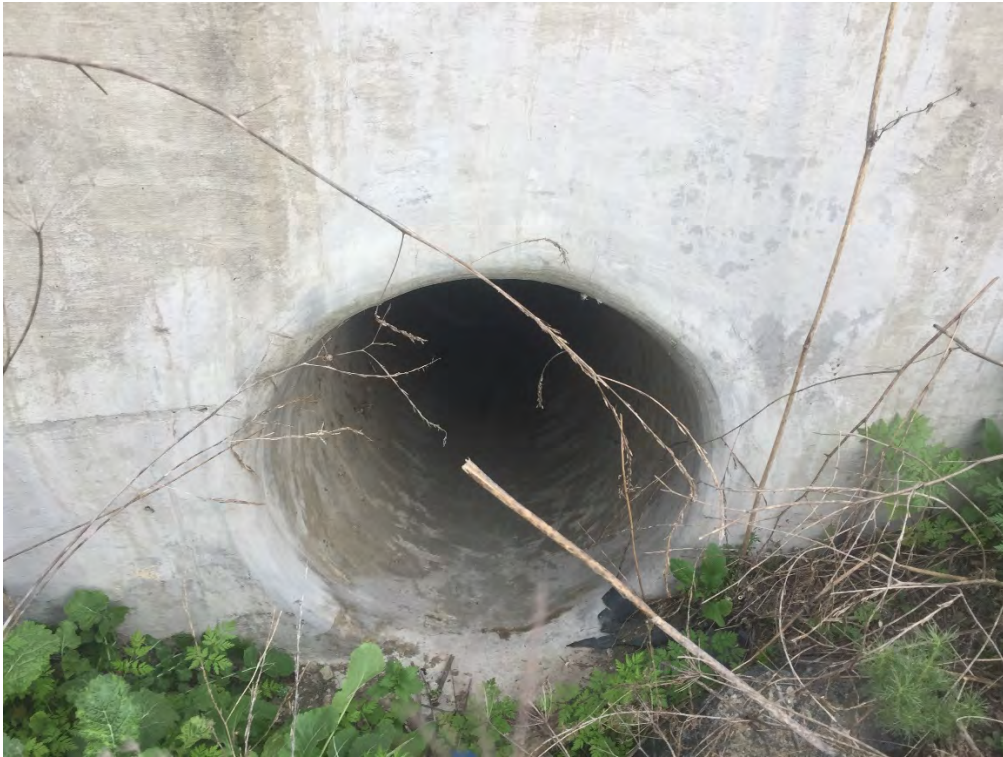
Photo 5: Culvert at the end of Feature A; facing north.
