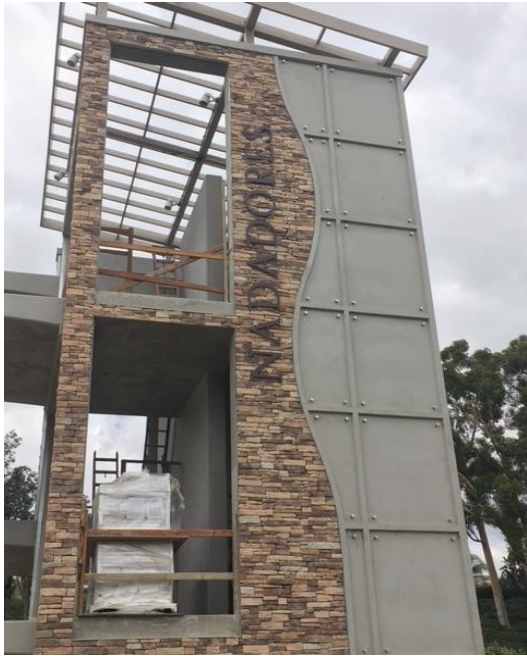
Stone Complete and signage beginning To be installed.
