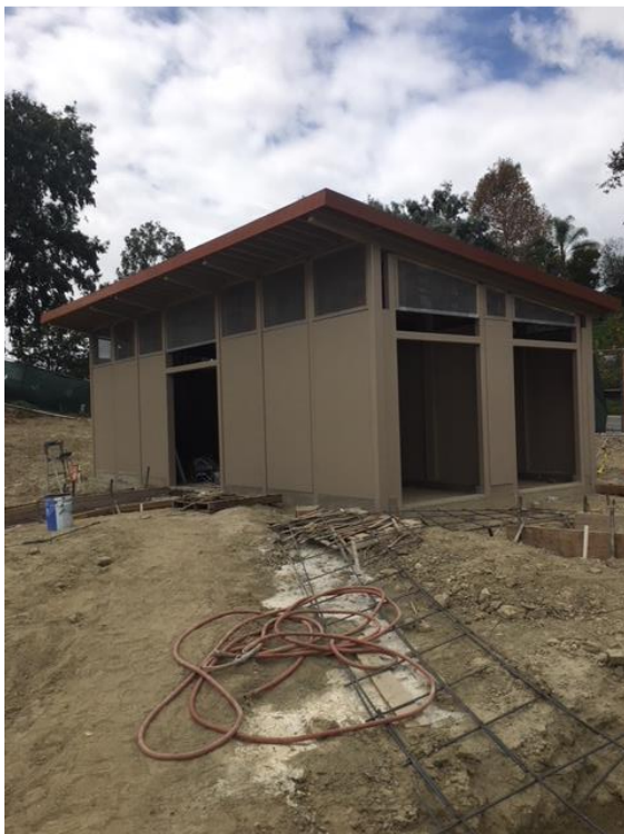
First Coat of paint on the Activity Pool Building.
