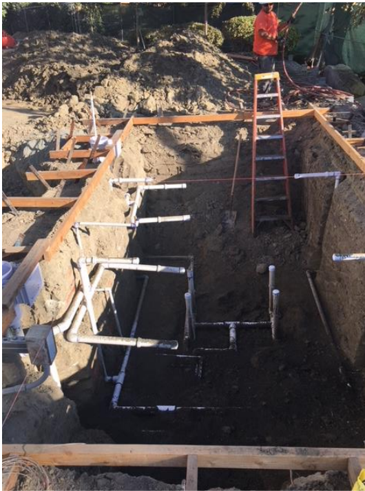
Plumbing for new warming pool/Spa
