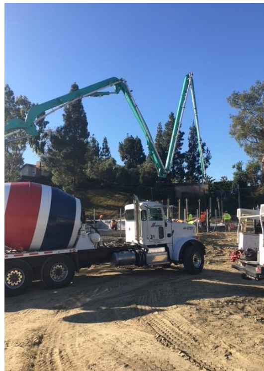
Pumping of Concrete for Pool Decking and shade cover footings.
