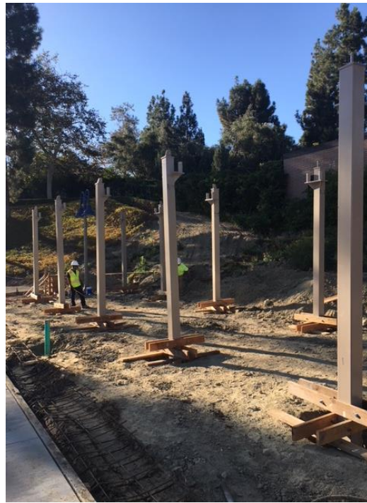
New shade Structure at Activity Pool.
