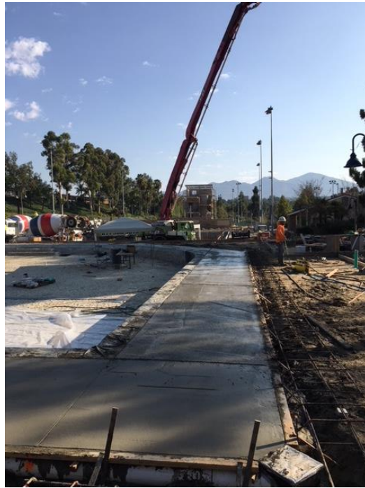
Activity Pool Decking formed and poured.
