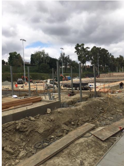
Swim Office Storage Area Fencing Poles
