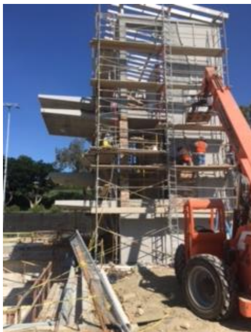
Stone being placed on the Dive Tower
