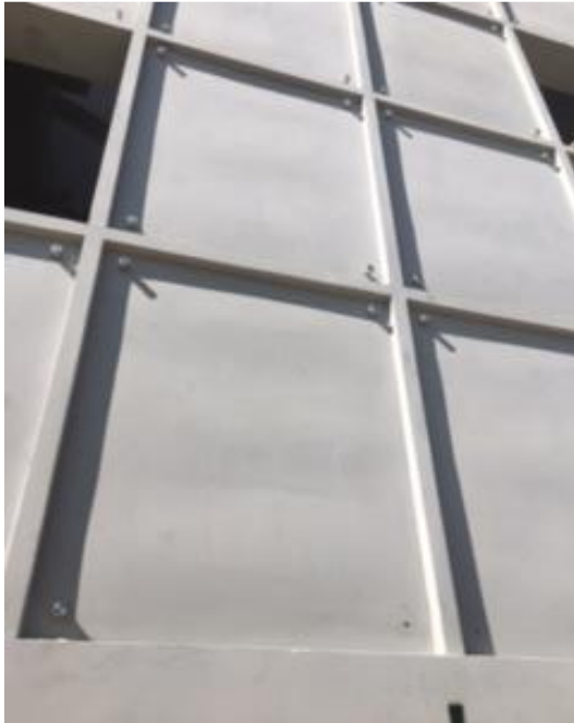
“Stand- Offs” for Tower Glazing Installed
