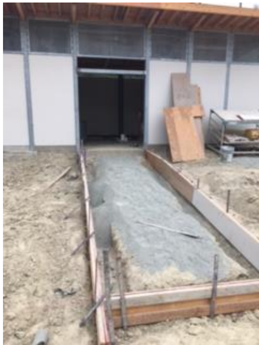
Activity Pool Pump Room Ramping
