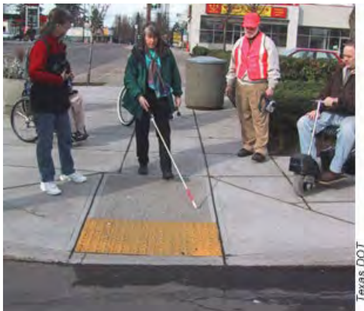
FIGURE 39: EXAMPLE OF TRUNCATED DOMES ON A PEDESTRIAN RAMP
