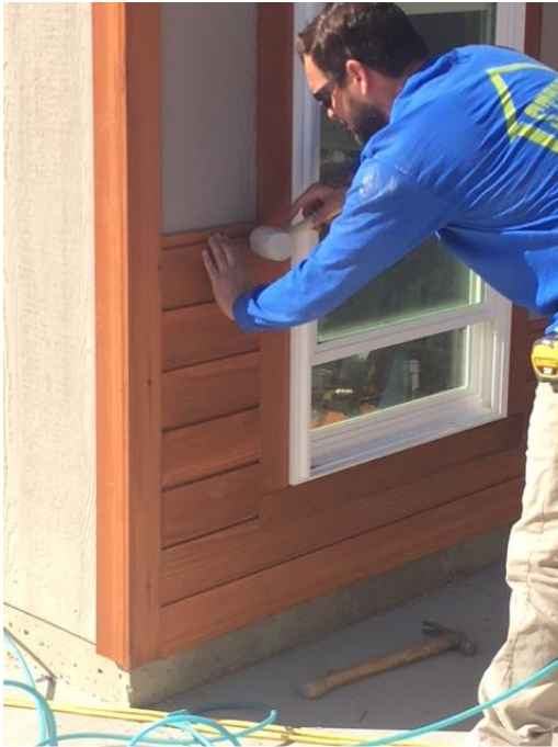
Dive Pool Office installation of siding
