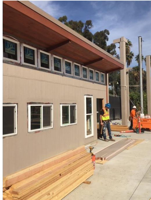
Dive Pool T&G installed on Building Eve
