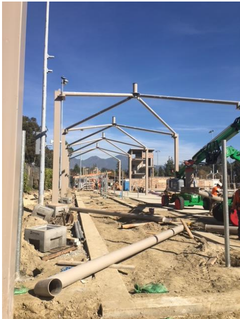
Grandstand Shade Structure Roof Support
