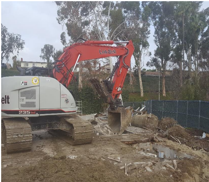
DEMOLITION OF EXISTING SPA
