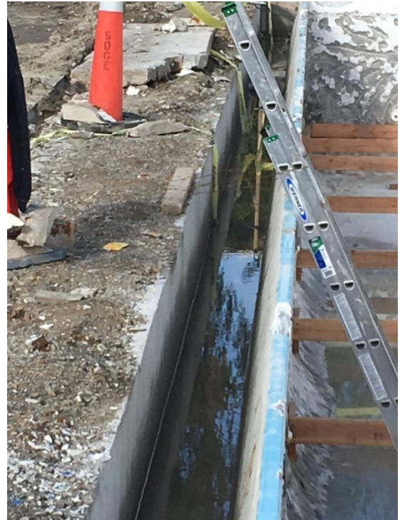
GUTTER AND LIP REPAIR UNDER WAY
