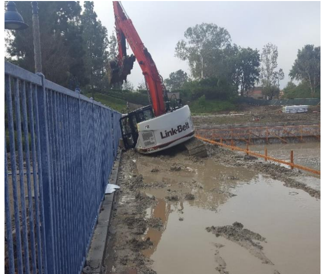
EXCAVATOR STUCK IN MUD AFTER STORM TRYING TO EXCAVATE AND KEEP PROJECT MOVING
